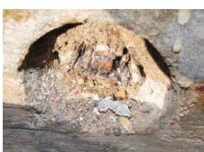
With standard grout plugs, the cementitious grout shrinks and becomes loose. Poor bond and/or poor quality mortar permits aggressive materials easy access to anchorage and prestressing steel. Precast grout plugs do not fill the entire void made by the pocket former, require complex installation procedures, and are very expensive.
