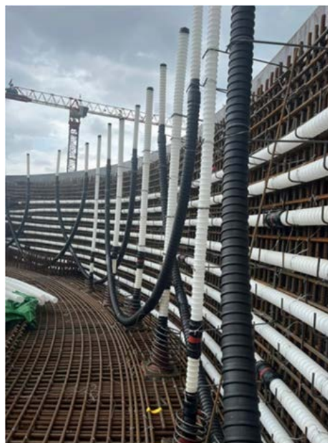
Fig. 5: Tank with GTI® plastic ducts for horizontal and vertical post-tensioning and GTI Tight Radius ducts for the loop tendons
